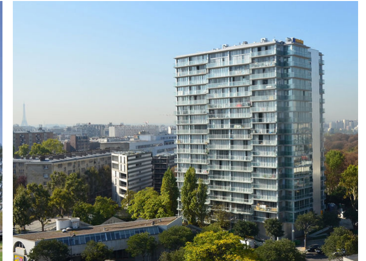
Refurbishment project at Tour Bois-le-Prêtre by Lacaton & Vassal Architectes
