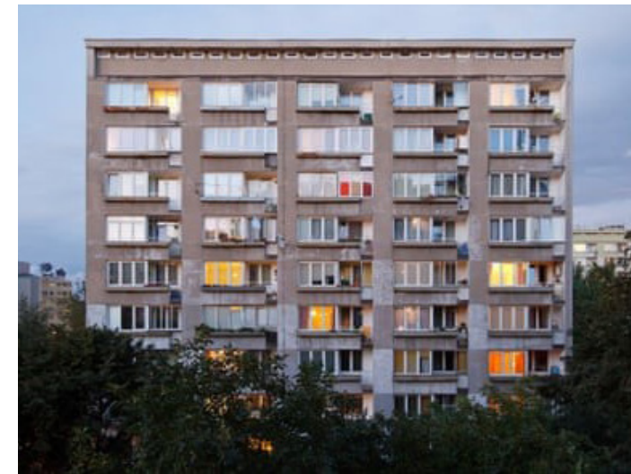
Refurbishment of soviet-era prefabricated building in the center of Warsaw
